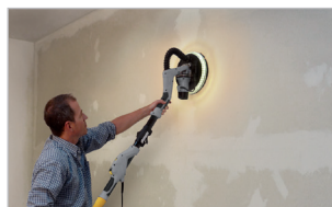
Eclairage rasant par LED LED grazing lighting
